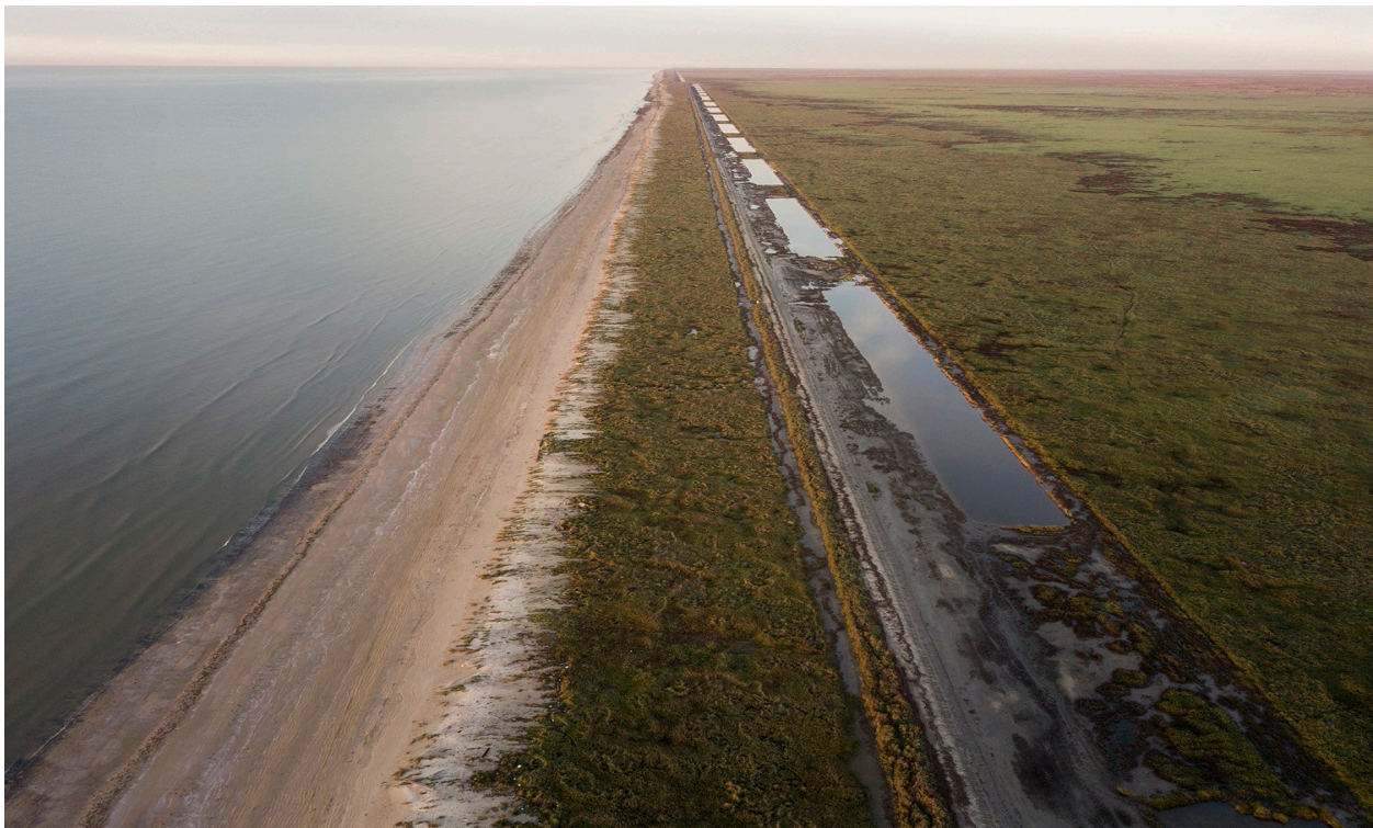
Figure 1-5: Constructed clay berm and beach nourishment at McFaddin National Wildlife Refuge
