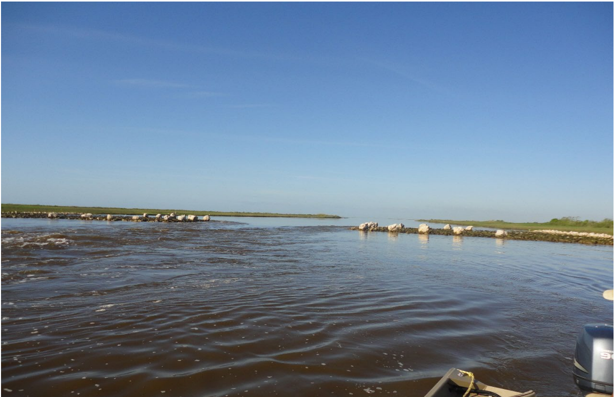
Figure 1-2: Completed Keith Lake Fish Pass Baffle Project
